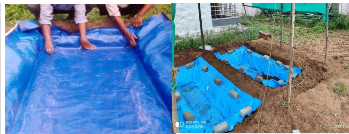
Polyethene sheet covered in trench
